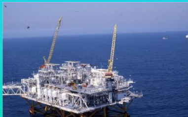
March 12, 1980 Platform Elly Installed.
